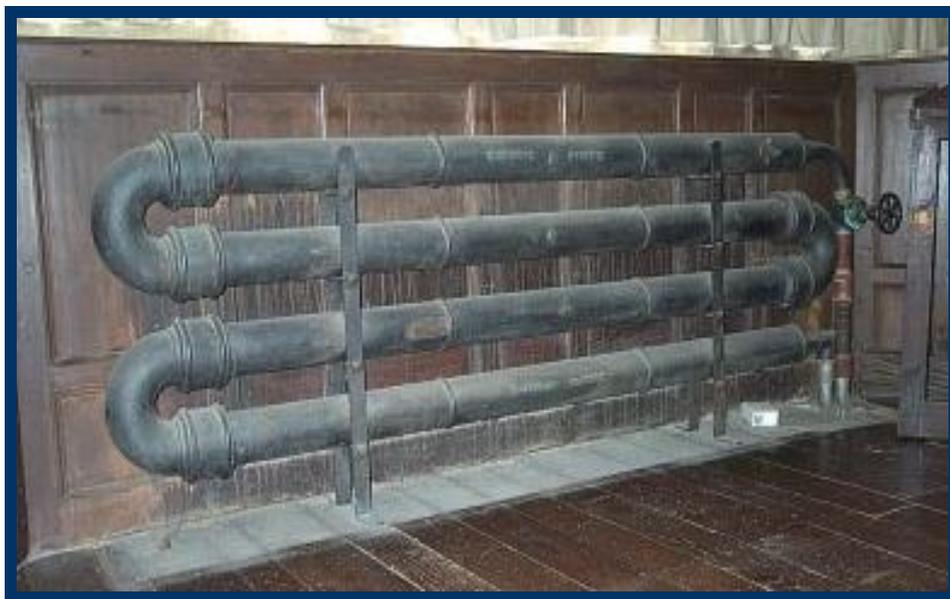
Cast iron pipework heating coil marked "W Sparrow, Martock"
