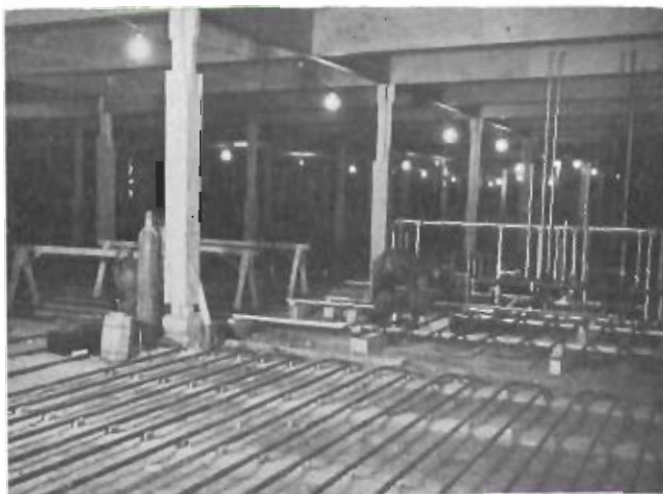
Fig. 4—Pipe coils in place before pouring concrete slab
