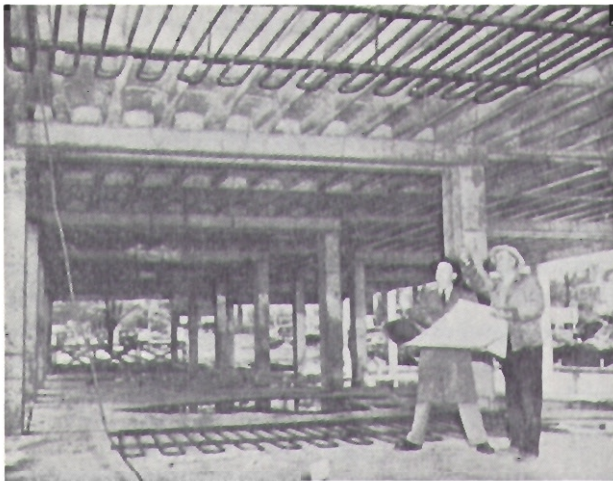
Fig. 2—Pipe Coils for Ceiling Panels
