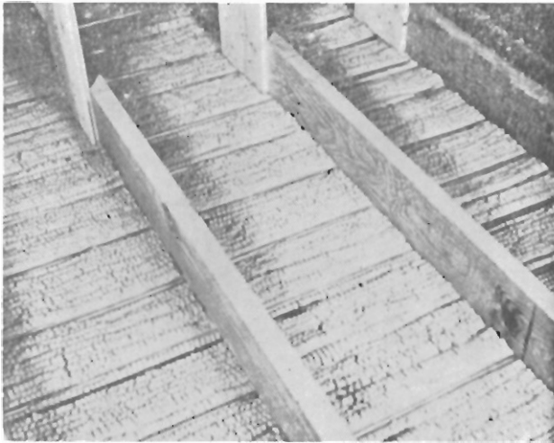
Fig. 6—Plaster in Contact with Tubes
