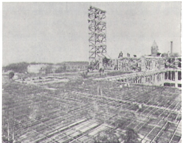
Fig. 4—Pipe Coils in Multi-Story Structural Slab
