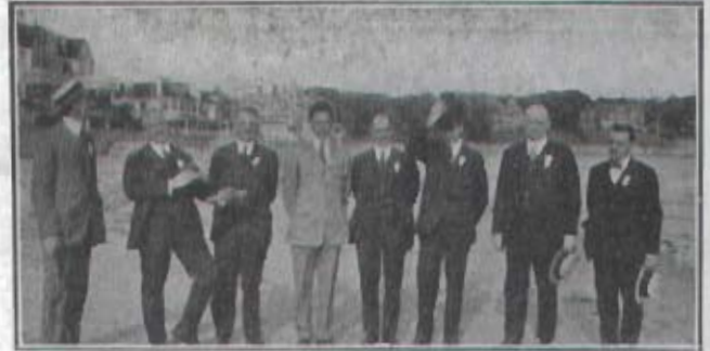
PRESENT AT CONVENTION OF HEATING AND PIPING CONTRACTORS
