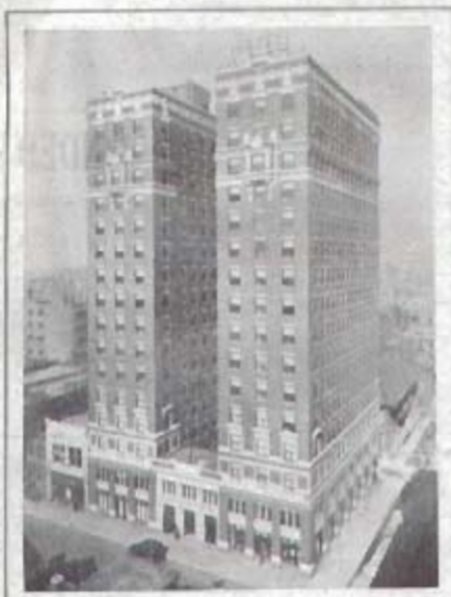
Hotel Wolverine, Detroit, Mich.: National Plumbing & Heating Supply Co., Chicago, Jobbers; W. G. Cornell Co., Plumbers; George H. Gottschalk Co., Architects
