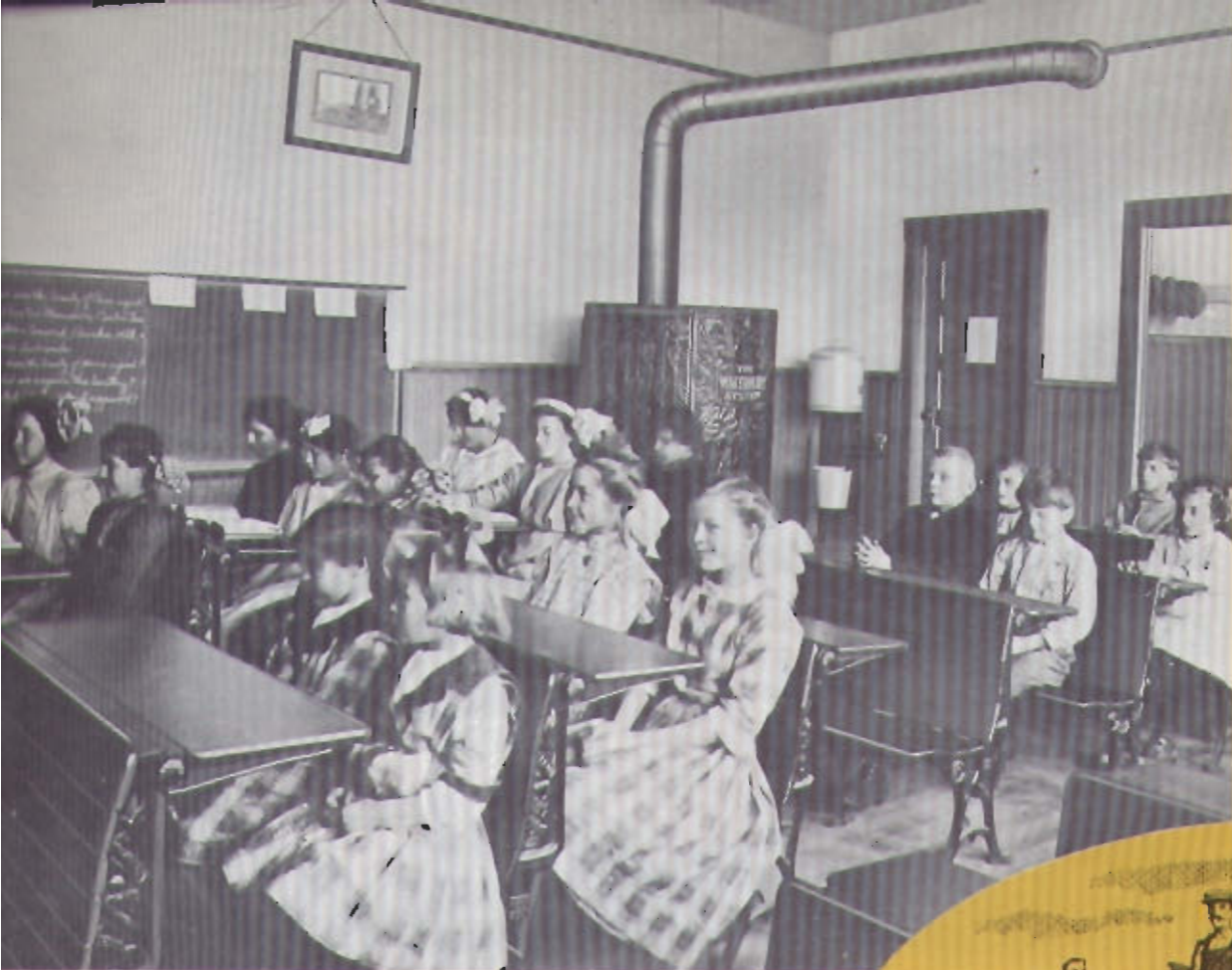
ONE ROOM SCHOOLS about 1910 were heated with "School Room" hot air heaters, considered to be the latest for health and comfort.
