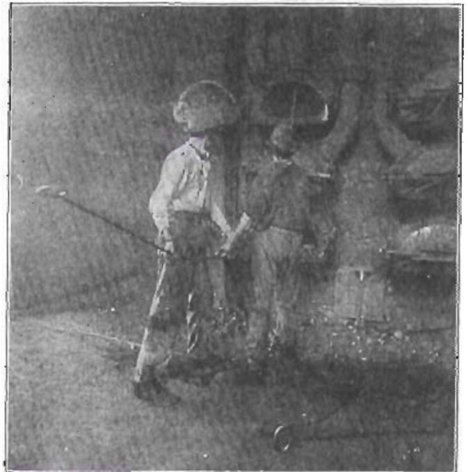
The Old Method of Discharging the Retorts
