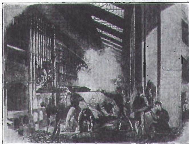
Retort House in Old Manhattan Gas Works
