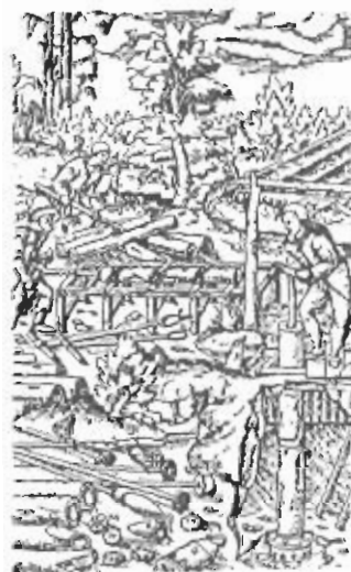
Boring Logs for Pipes Used in Early Days of the Gas Industry
