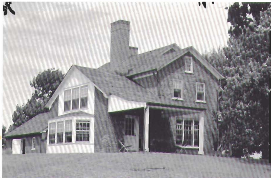
Installation of radiant heating, with Rayduct steel pipe, was one feature of extensive renovation in this residence at Washington, Conn.
