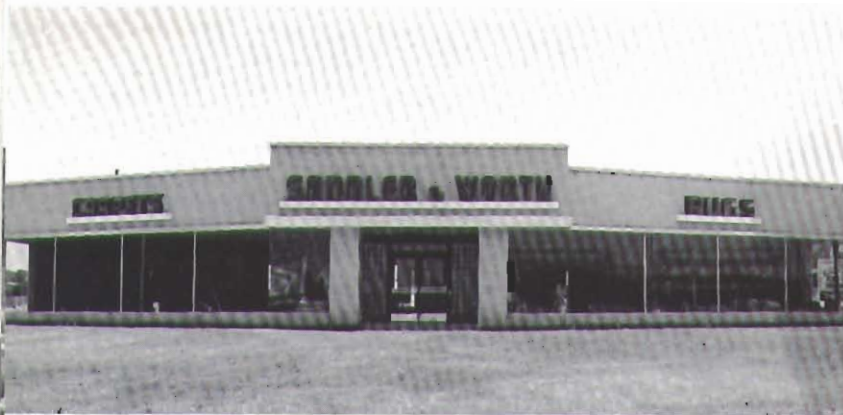
Rug showroom on busy Route 29, at Springfield, N. J., has floor-type radiant heating, using Rayduct. Below: Interior view of showroom shown above.
