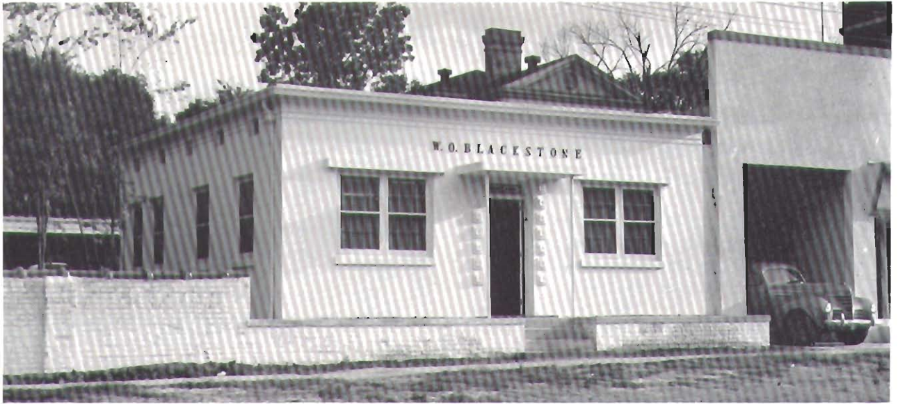
This building at Columbia, S. C., housing an office, garage and showroom, is equipped with Rayduct floor coils.
