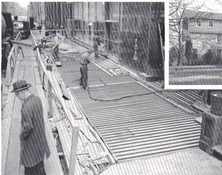
Left: Sidewalk installation, New York.
