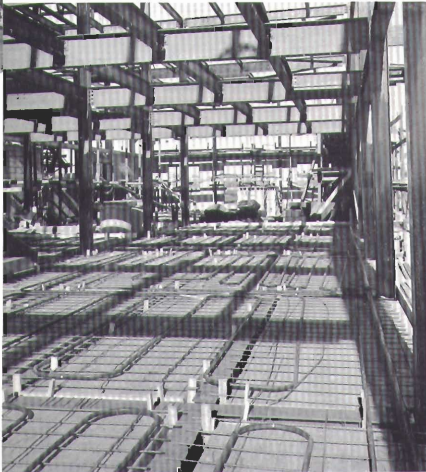
Radiant-heating system being installed in Bethlehem Steel Company office building, Cambridge, Mass. In completed building, employees work in comfortable surroundings.
