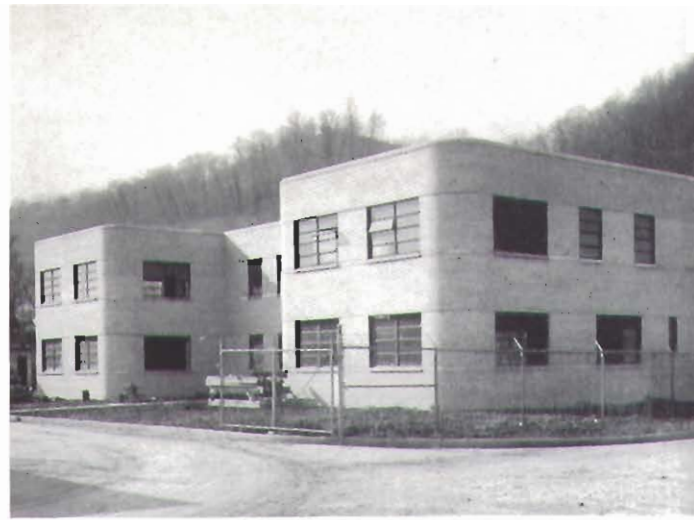
This attractive administration building at Wheeling, W. Va., has Rayduct floor piping in both first and second stories.
