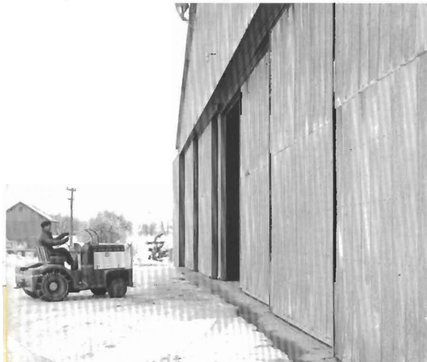
Warm water, circulating through Rayduct piping buried in concrete under hangar doors, keeps ice from forming, and makes doors easy to open.
