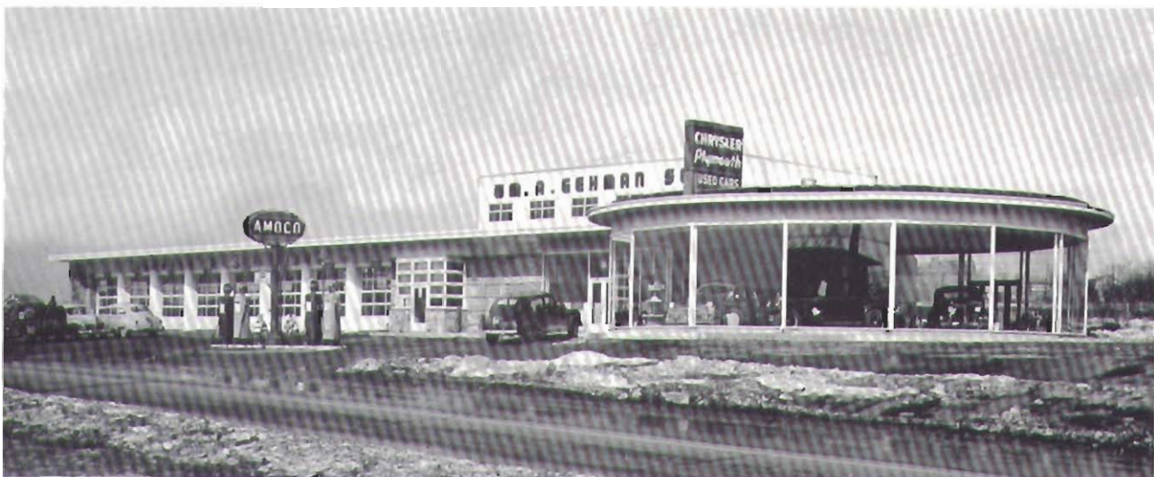
This garage and automobile salesroom, located in Emmaus, Pa., is heated by means of a radiant-heating system, using Rayduct.
