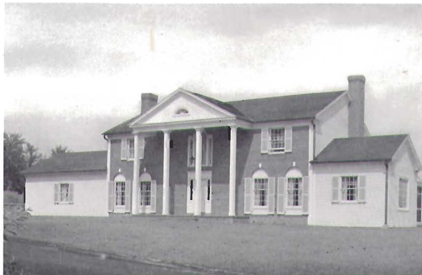
A radiant-heating system, with Rayduct steel pipe, is one of the features of this new residence at Litchfield, Conn.
