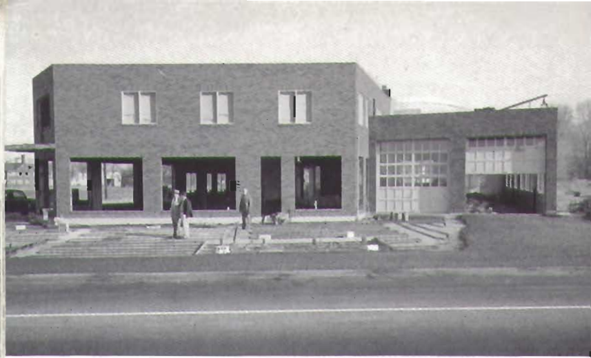
In addition to apron piping, Rayduct is used in both stories of this automotive building at Quakertown, Pa.
