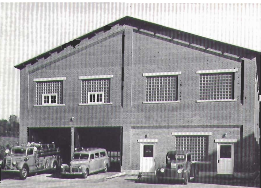
Two-story fire house and service building at the Steelton, Pa., plant of Bethlehem Steel Company, equipped with a Rayduct radiant-heating system in both stories.
