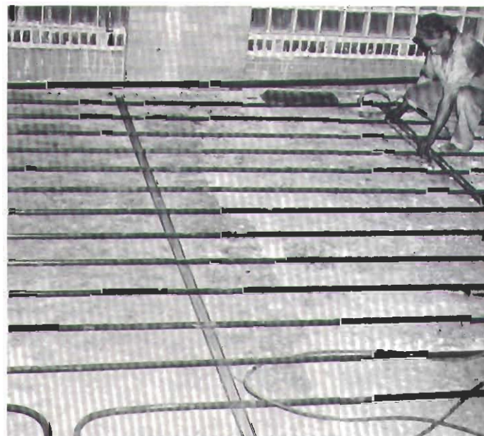
Warm water, circulating through Rayduct piping buried in concrete under hangar doors, keeps ice from forming, and makes doors easy to open.
