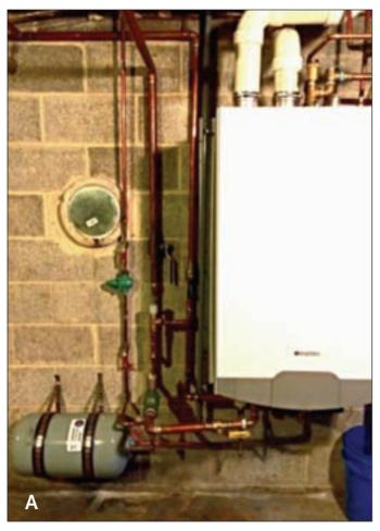
When no call for heat exists, the supply piping from the boiler to the zone valves is completely isolated from the expansion tank. During a call for heat, this section of piping is full of hot water.
