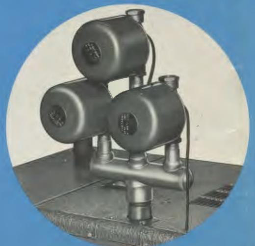
Available on all 'Donobilt' Boilers — 2 and 3 zone valve sets, mounted on header and wired at factory.
